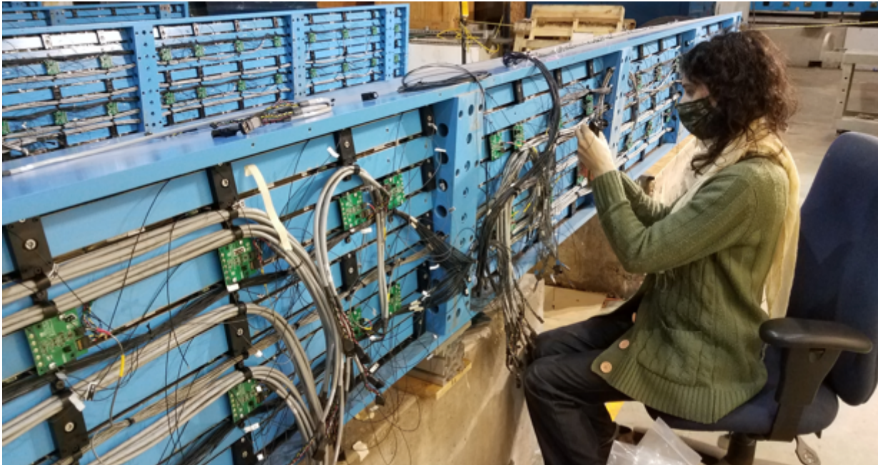
▲ Fiber-optic cable installation by Veronica Canoa Roman before electronics boxes are installed
